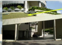
Artificial landscape sheltering parking space from sunlight
